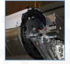
A reduced drive chain hoist for smoother operation is standard on all door sizes over 10'0" x 10'0".
